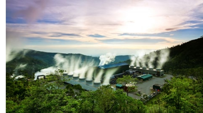
Mahanagdong Geothermal Project (Ongoing)
